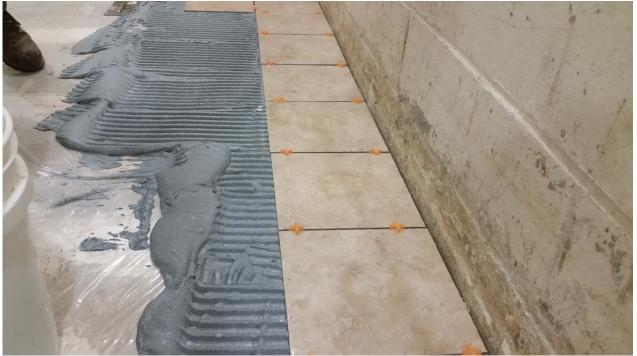
Figure 3 – Mortar and tiles partially installed over concrete slab
